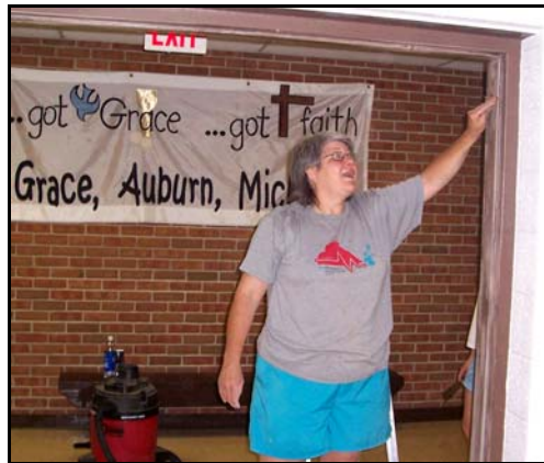
Gayle Woods sanding down the door frame.
